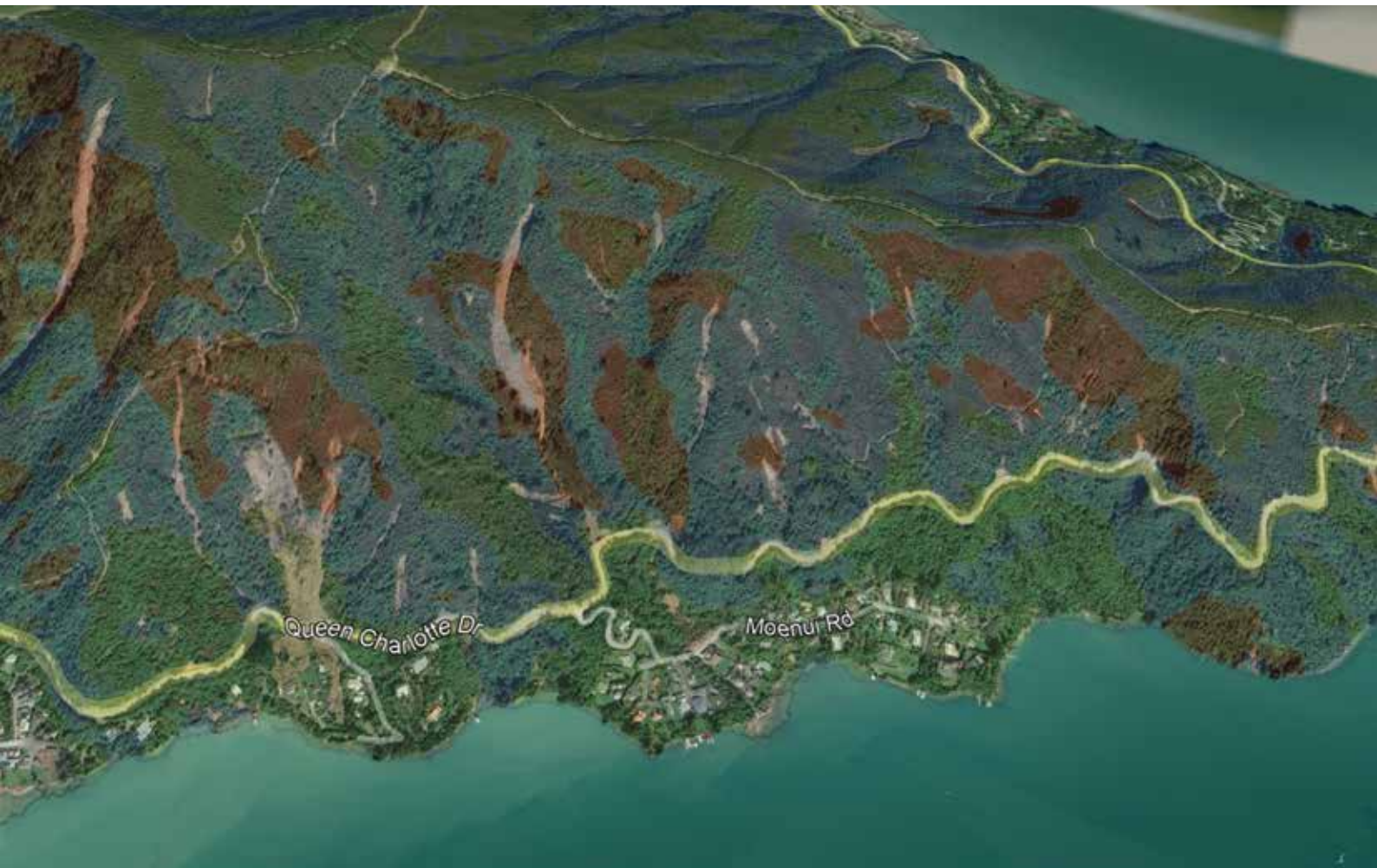
Figure 3: The area between Belvue Bay Road and Moenui Road on Queen Charlotte Drive showing multiple landslide scars after the July 2021 rainfall event. The coloured shading shows slopes: <26 degrees (green), 26–35 degrees (pale) and >35 degrees (red). The ESC maps the entire area as green (low erosion susceptibility). Source: Google Earth and unpublished slope analysis by the author and David Palmer (Scion)
