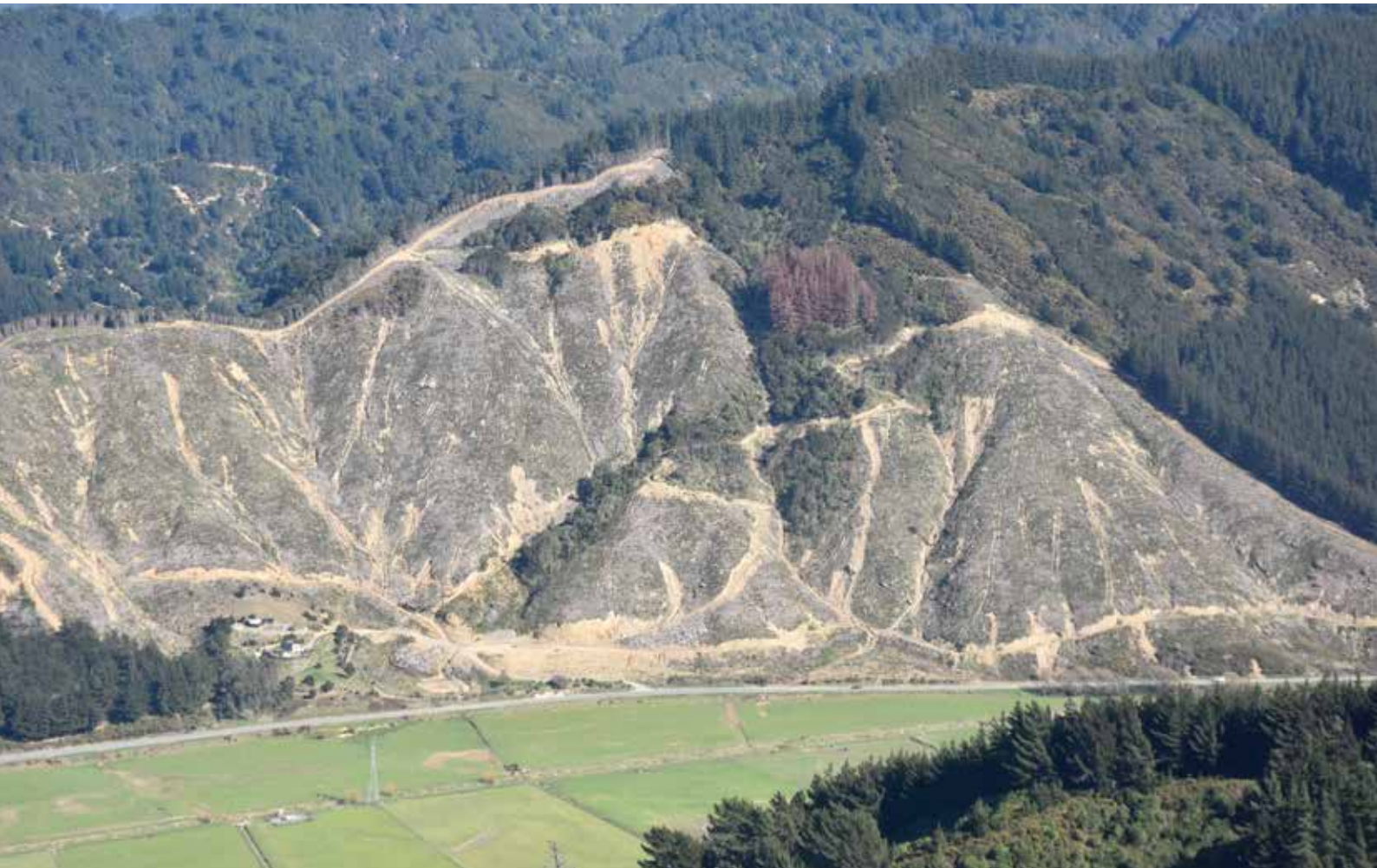
Figure 2: Landslides from a harvested forest in North Marlborough in 2022. The landslides impacted the state highway (SH6) at the bottom of the slope. Source: Matt Oliver, Marlborough District Council
