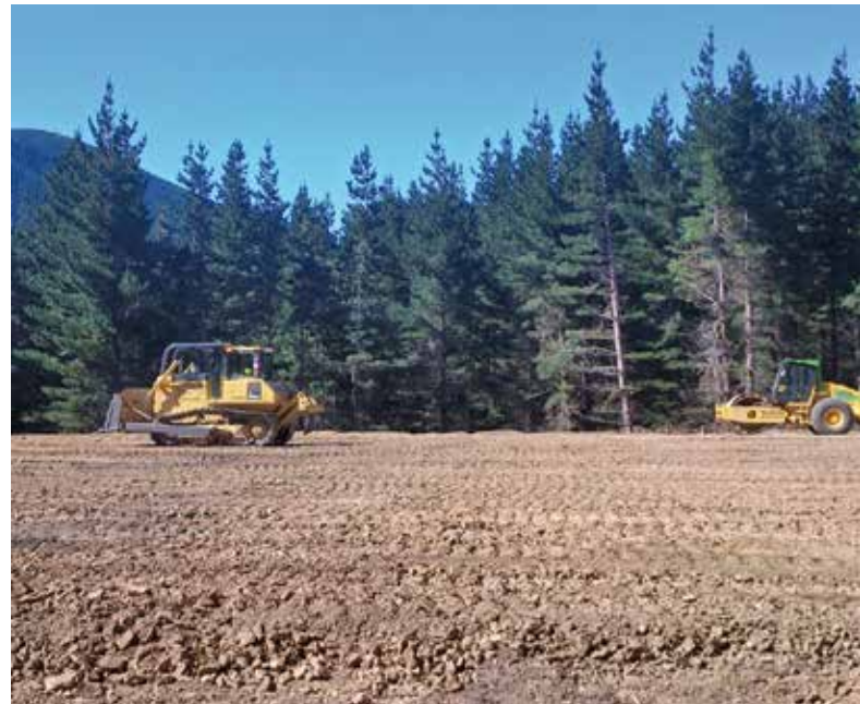
Summertime landing construction in Canterbury. Compaction involved track rolling the landing with a Komatsu D65 EX bulldozer (left) prior to vibratory rolling with a Sakai SV512TF (right)
