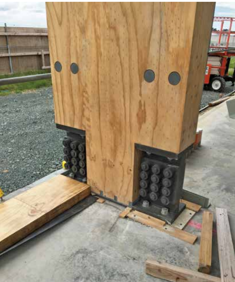
1200 x 300 mm LVL column with two RSFJs connected at the base building project conducted for Airways NZ rather than Nelson Airport.
