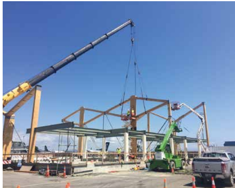
Erection of pre-assembled 'diamond' beams and columns
