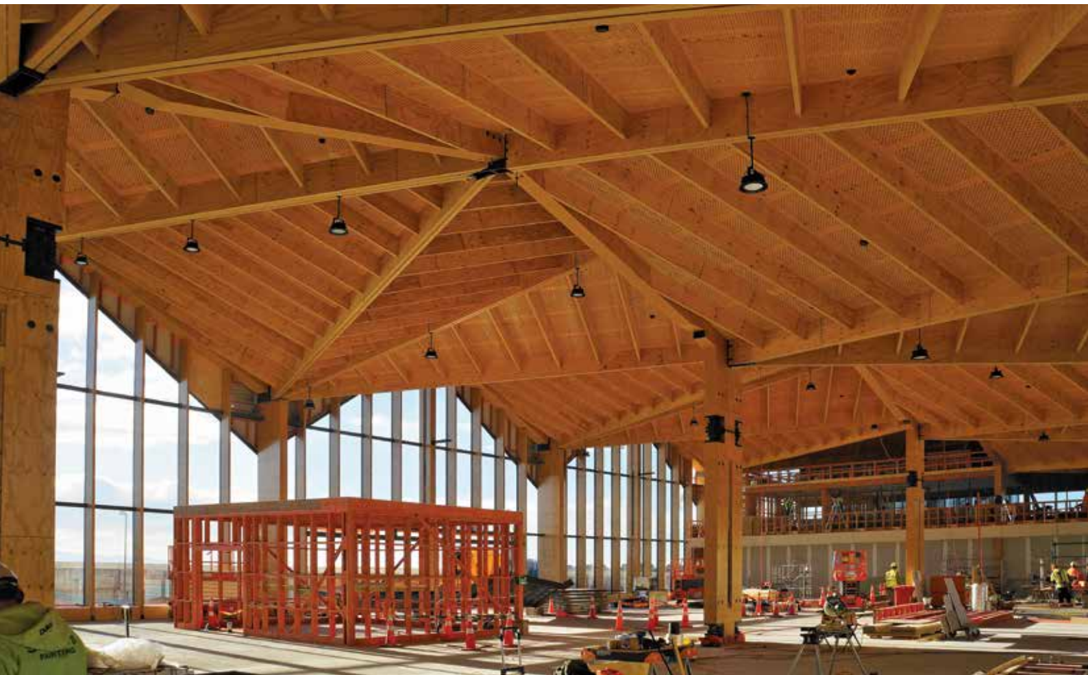
Engineered timber in the Nelson Airport Terminal under construction. Photo courtesy of David Evison
