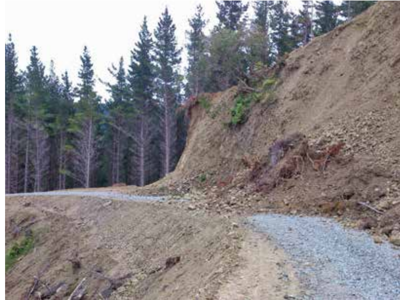
A cut slope on a newly-constructed road that has slumped following a rainfall event in Gisborne
