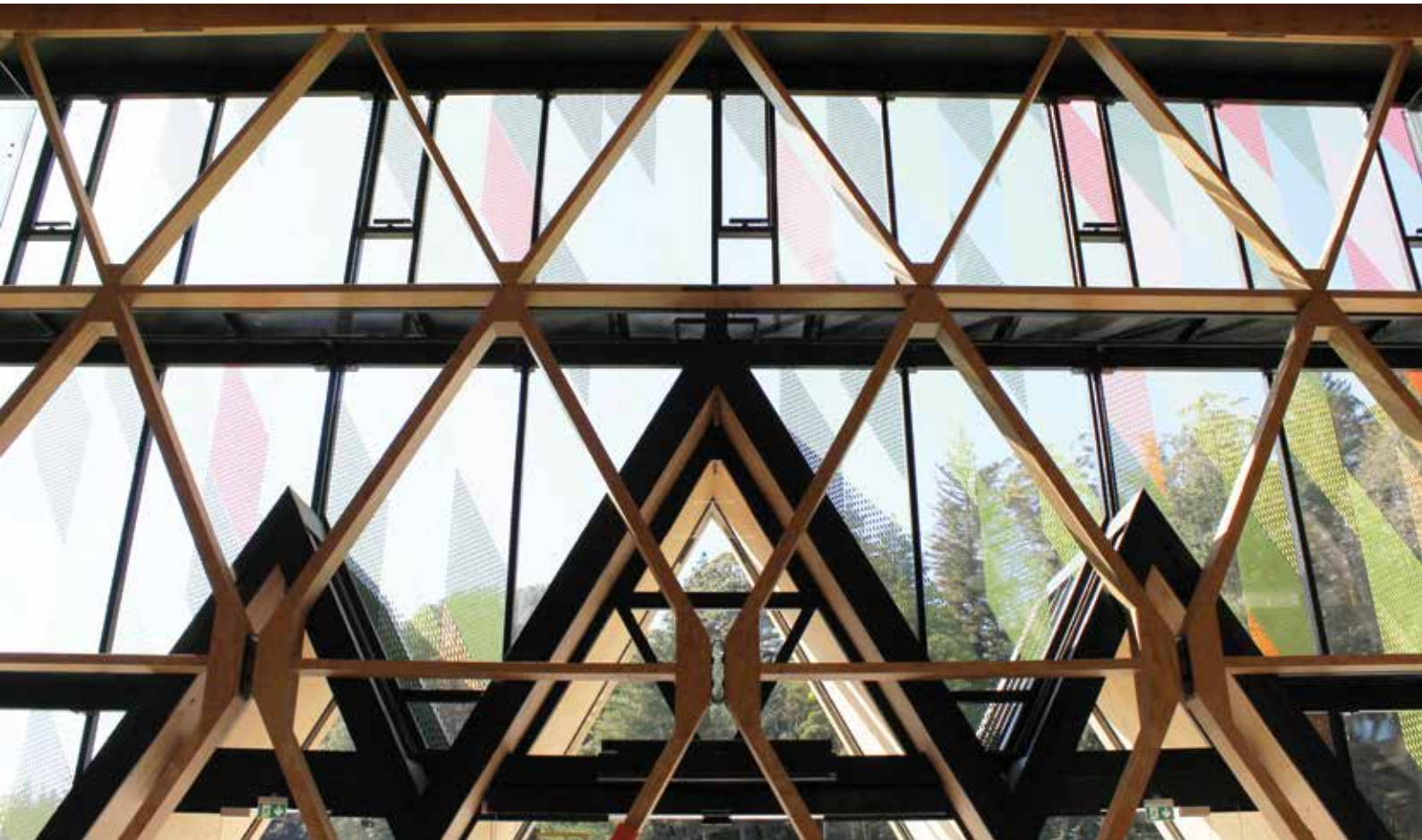
Timber buildings are carbon stores. Scion's new building constructed around diagonal grids of laminated veneer lumber (LVL) is storing approximately 0.418 Mt of CO 2 -e, the equivalent to the emissions from 160 return flights from Auckland to London
