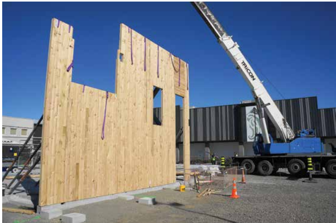
Erection of CLT panels, Hornby Club site, 10 September 2019
