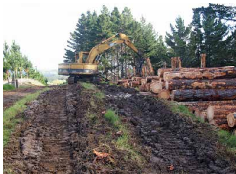
Load out site on ridge top beside main logging road
