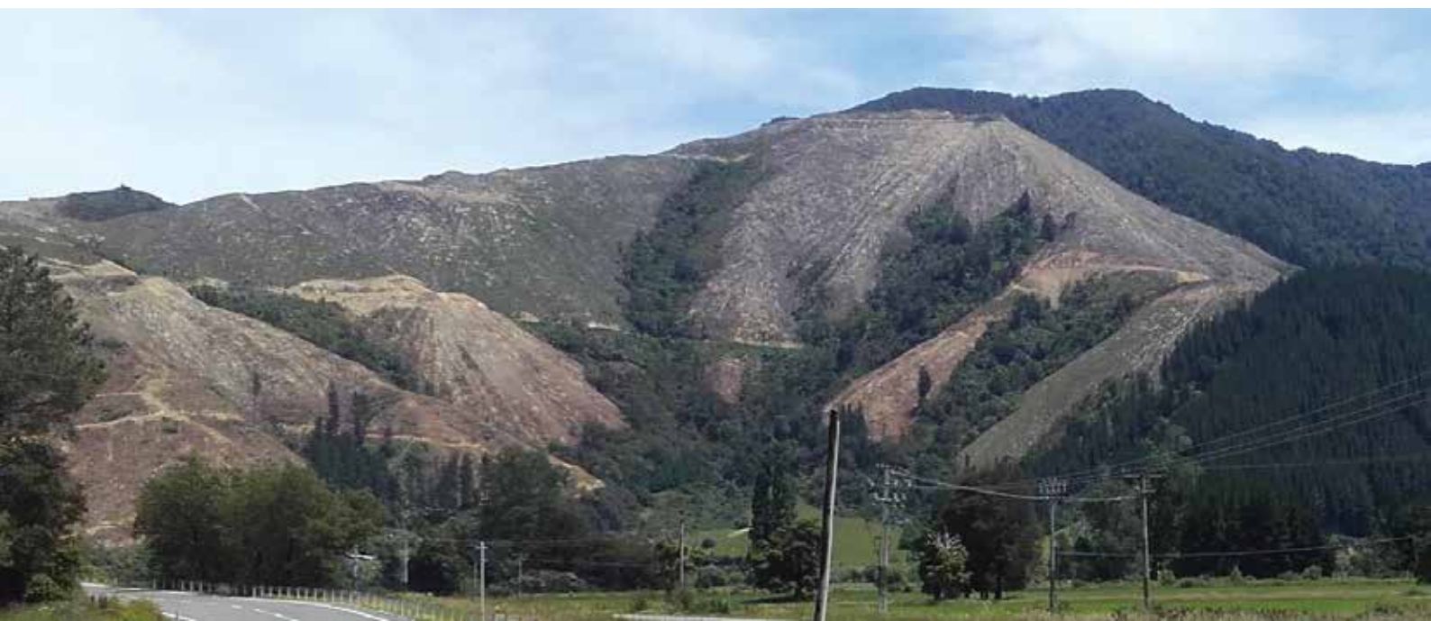
Example along the lines of what a replanting management plan aims to achieve. Note the retention of mature indigenous forest in steep erosion-prone gullies and faces and careful placement of roads and landings, Havelock, 2016. This operation had issues with woody debris left in a waterway out of view
