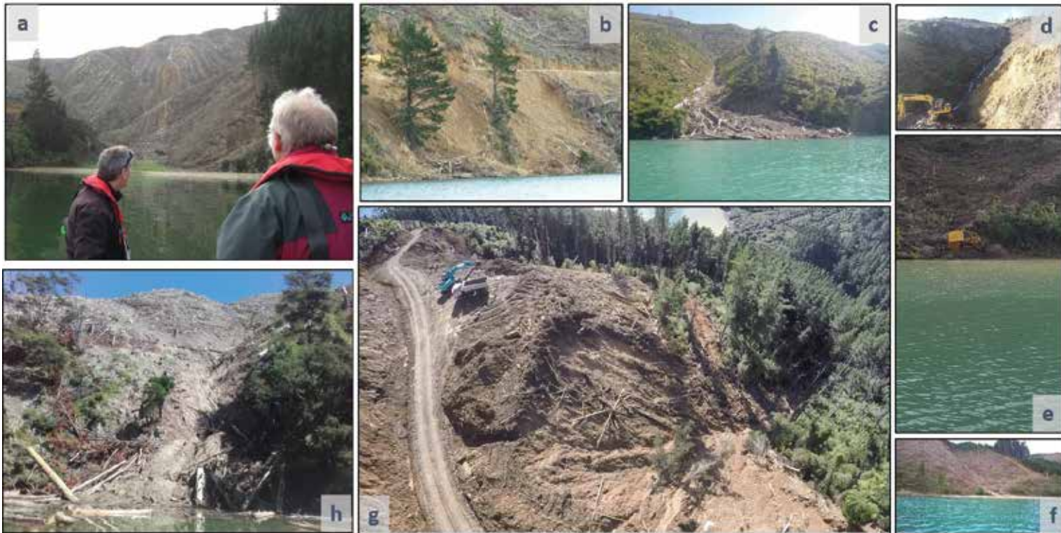
Figure 1: Relatively common issues from forestry earthworks and harvesting in the Marlborough Sounds: (a) Log-scoured runnels by inadequate lift from a cable hauler cable on a ridge top and pulling across slopes, Port Underwood, 2016; (b) Batter slump, and fill failure from logging road into Pelorus Sound, 2012; (c) Debris flow post-harvest, Pelorus Sound, 2011; (d) Post-harvest slope failure and top of debris flow, which smothered an estuary, 2015; (e) Bulldozer mishap above the shoreline Tory Channel – note sediment discoloured waters close to shore; (f) Harvesting to the shoreline, vulnerable to sediment run-off, Tory Channel, 2016; (g) Landing failure from inadequate water controls and poor construction resulted in debris flow down a forested creek, with sediment discharge into Pelorus Sound, 2017; (h) Debris flow with logs and soil after Cyclone Gita, Port Underwood, 2018. Photos: MDC – except (e) courtesy of Peter Beech
