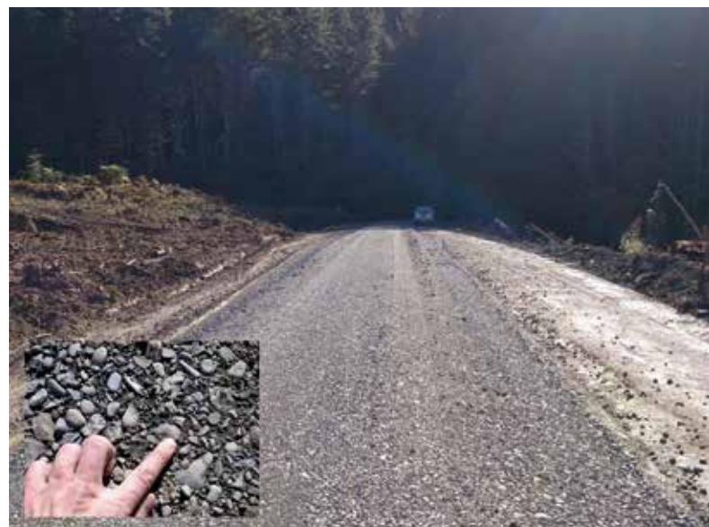
Newly-constructed secondary road on the East Coast
