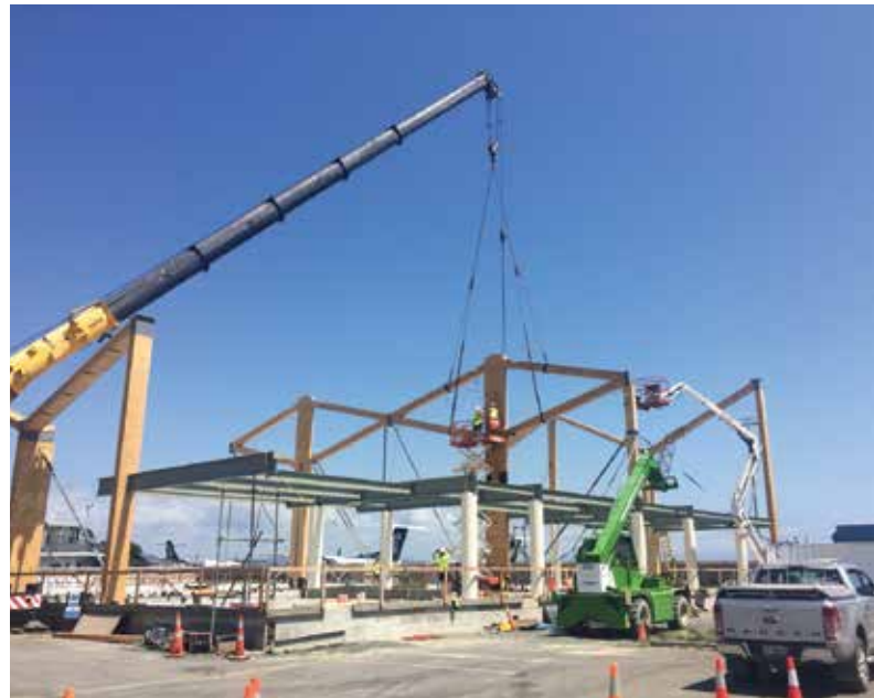
Erection of pre-assembled 'diamond' beams and columns
