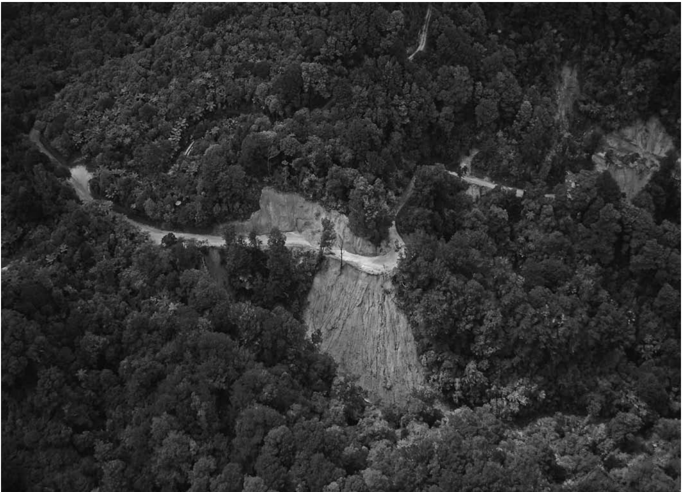
Studies worldwide have shown that roads increase landslide erosion by two orders of magnitude compared with undisturbed forest land. Totaranui Access after the December 2011 storm. Photo courtesy of Gerry Draper.
