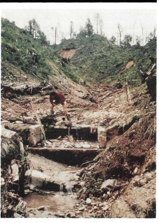
An extreme debris flow event demolished the stream gauging station and sediment trap in a recently logged experimental catchment at Maimai, north Westland. The debris flow accounted for a large per cent of the total sediment yield from this catchment over the first three years after harvesting.
