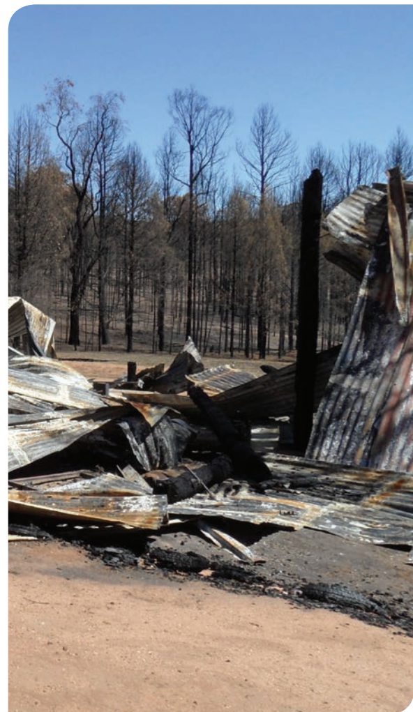
Burnt infrastructure Coonabarabran 2013 (photo: Dr Margaret Kitchin).
